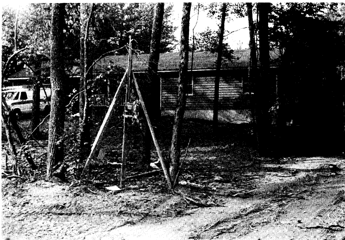
Fig. 2. Builders are aware of the increased sales price commanded by houses on wooded lots, and so have abandoned the practice of clearing all trees from a lot before construction begins. Only time will tell whether the trees remaining on this lot will survive the numerous stresses and abuses they suffer during the construction process.
